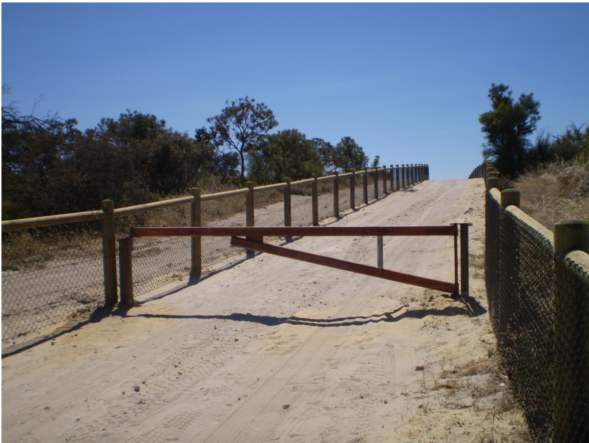
Plate 1: Example of access control fencing.
