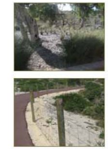
conservation / access control fencing
